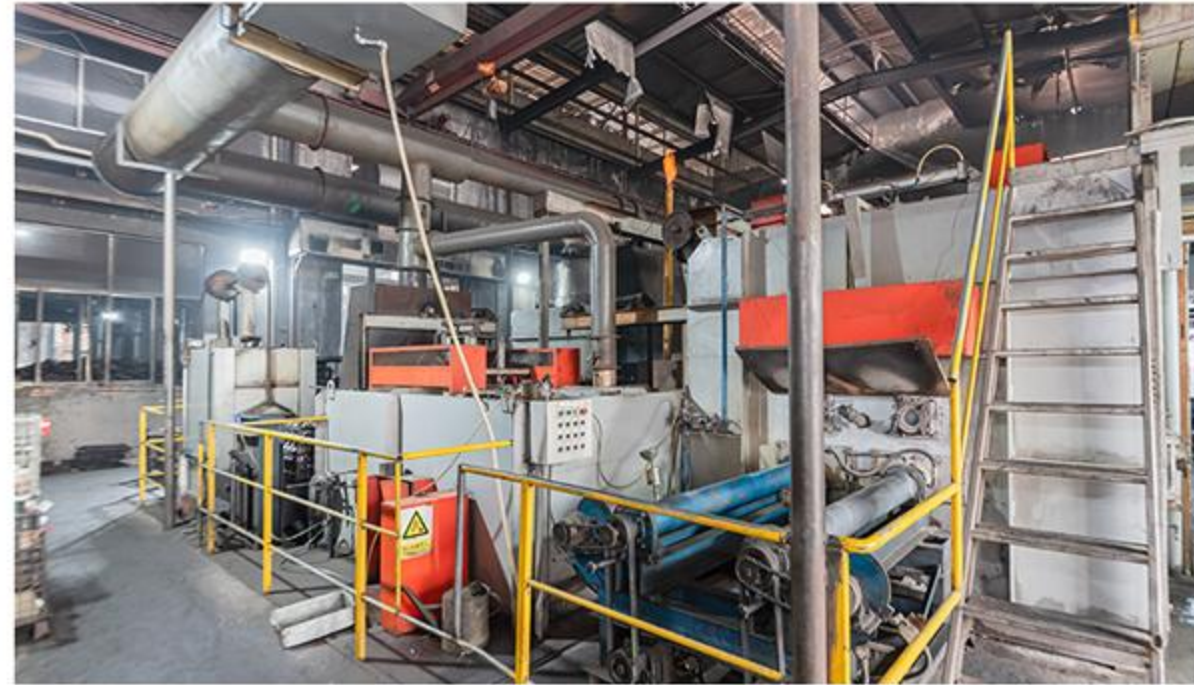
HEAT TREATMENT WORKSHOP
